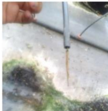
Gambar 4. Pengecekan selang drip
